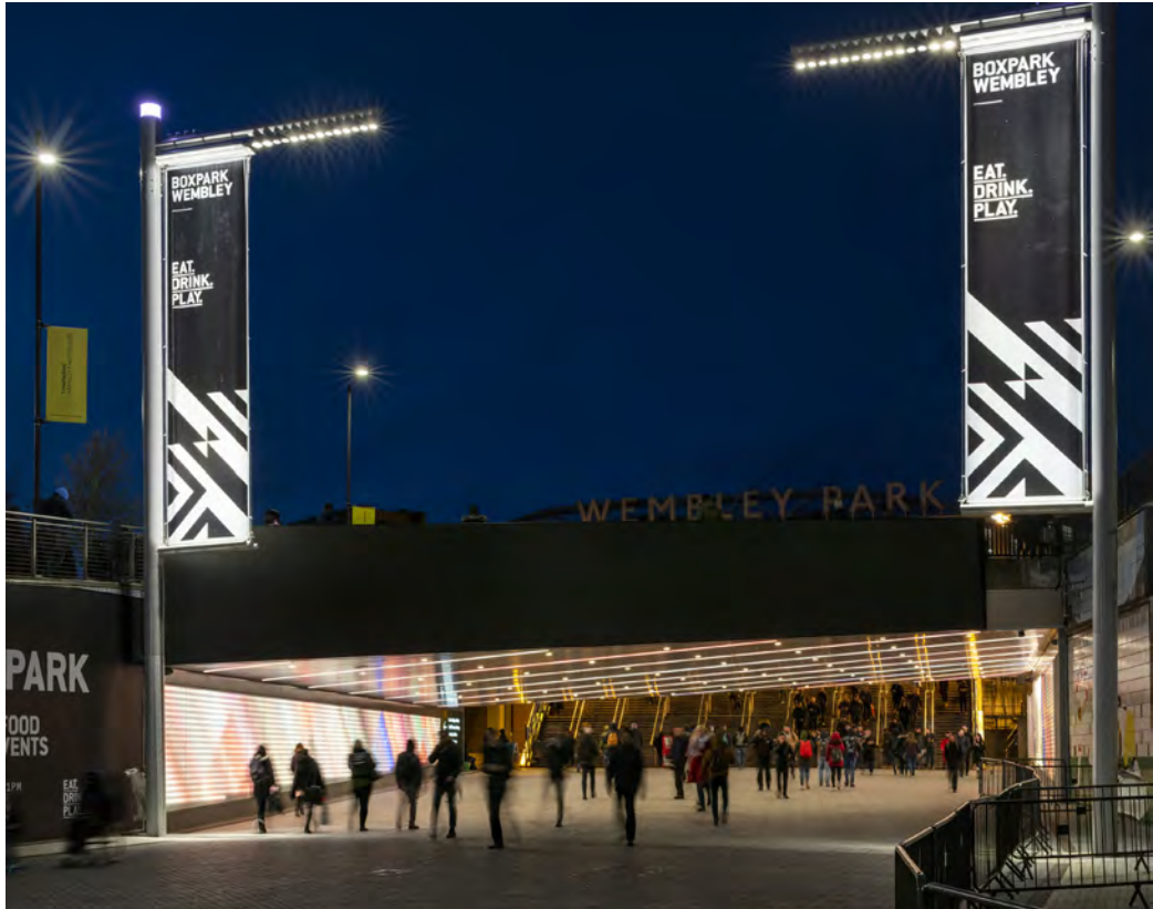
The optic that controls the downlighting to the banners also delivers rhythmic pools of light beneath each column. Photo: © James Newton
