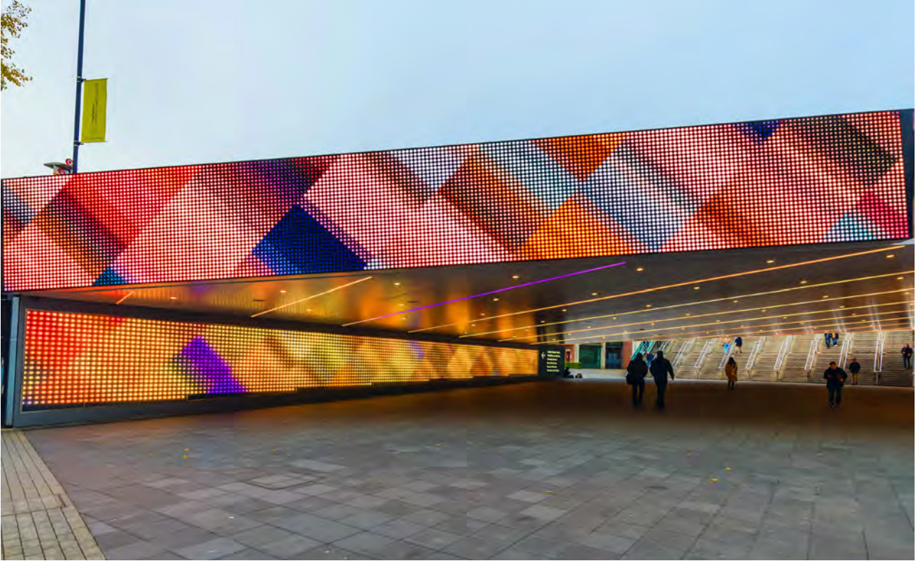
Low resolution screens and dynamic lighting slots allow content from the media screens on the fascias to appear to flow into the underpass. Photo: © Chris Winter
