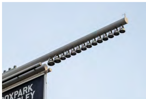
Each of the projector types has a unique optic, selected based on detailed lighting calculations and testing. Photo: © James Newton
