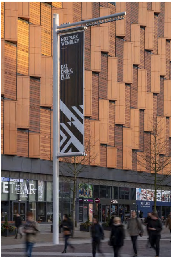
Their immense technical infrastructure means that each column can support up to one tonne of equipment, allowing digital banners to be installed in the future for live content and updates. Photo: © James Newton
